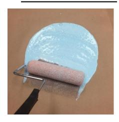
Keep the roller wet - Throughout the application process. For reference the installer should be able to scrape this much adhesive out of the roller. (See Photo left)
