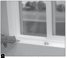
Apply 1-inch balls of polyurethane construction adhesive 3 inches from each end and 6 inches on center of the sill area.
