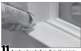
Apply a bead of caulk in the joints between the sill and the window, and the sill and the drywall. Smooth the caulk with a wet finger. Occasionally, the butt-cut ends will have voids. These voids can be filled with an all-purpose adhesive caulk.
