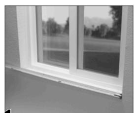
Measure the width of the window opening from jamb to jamb.
