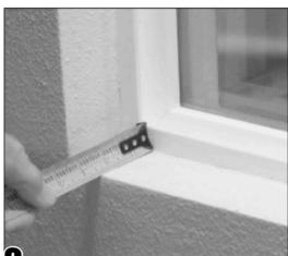
A Measure the depth of the window opening in three places (each end and the center). Note the largest of these dimensions.
