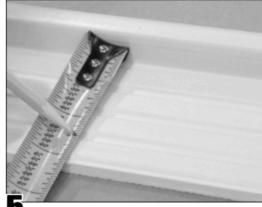
Mark the depth (the largest dimension from step 2) on the back of the sill, starting from the lip of the sill.
