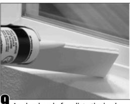
Apply a bead of caulk to the back edge of the sill.
