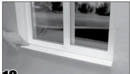
Insert the sill at a slight angle making contact with the window, then pivot the sill down in place.
