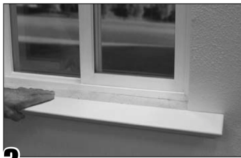
3 Align the center of the sill with the center of the window.
