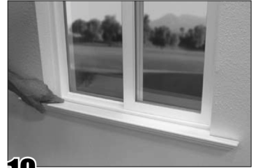
10 Insert the sill at a slight angle and making contact with the window then pivot the sill down in place.
