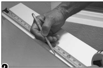
2 Measure and mark the center on the back of the sill.
