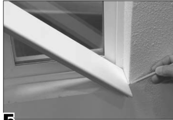
5 Insert sill into the window opening at an angle (as shown). Make sure the back of the sill is butt up against the window frame. Mark the depth of the window opening on the sill.
