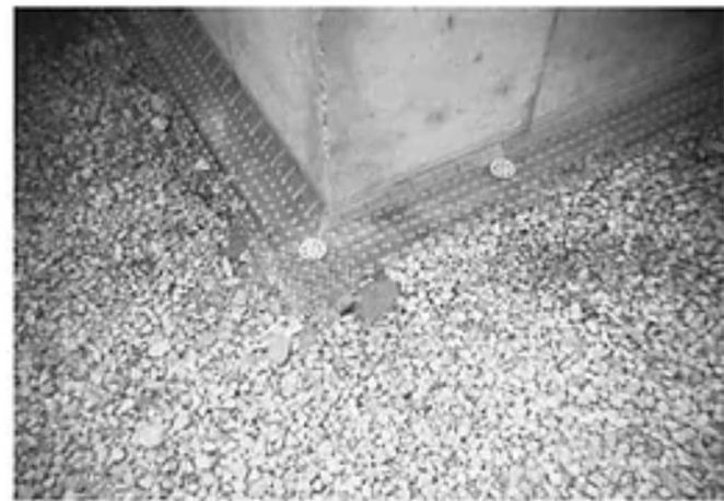
Inside corner installed
