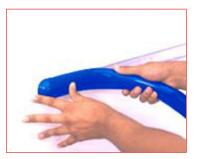
**2a. Flexible Top:** Butt end of the vinyl top against end/corner cap. While applying pressure with your thumb + forefinger, bend back vinyl top so that vinyl legs are positioned within the base grooves. Roll vinyl top over full length of base, then tap with rubber mallet to ensure vinyl is securely locked into the base.
