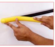
**2a. Flexible Top:** Butt end of the vinyl top against end/corner cap. While applying pressure, bend back vinyl top so that vinyl legs are positioned within the base grooves. Roll vinyl top over full length of base, then gently tap with rubber mallet to ensure vinyl is securely locked into the base.
