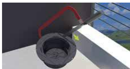
1. Cut one side of the pedestal.
