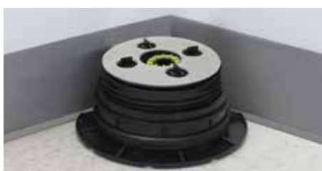
2. Assemble the pedestal and position it in the corner.
