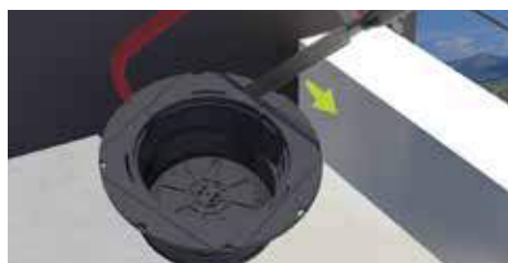
13. Cut one side of the pedestal.
