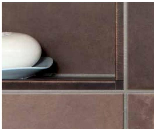
**QUADEC** square-shaped profile and corners applied to tile edges and outside corners of the shower including the shower bench and niche, and used to finish the tile base. **DILEX-AHK** cove-shaped profile and corners used to create a smooth transition between the walls and floor.
