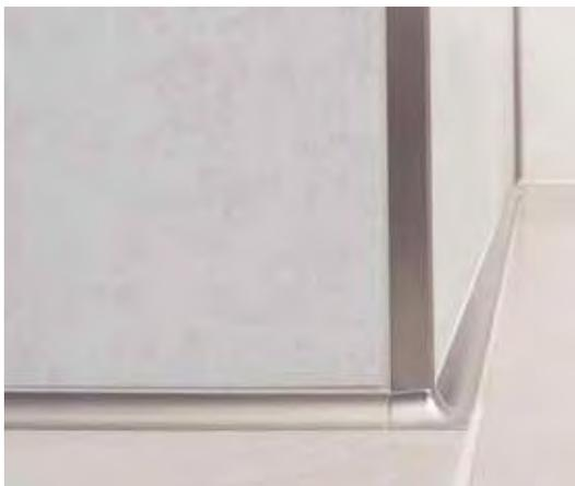
**QUADEC** square-shaped profile and corners used to finish the tile edges on the wall. **QUADEC-FS** double-rail edging profile used to frame the mosaic insert in the wall. **DILEX-AHK** cove-shaped profile and corners used to create a smooth transition between the floor and wall.
