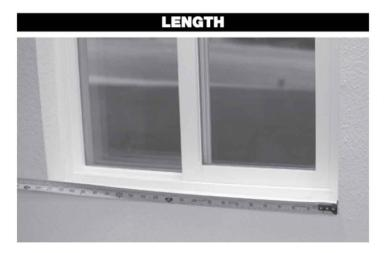
Measure the width of the inside jamb of the window opening.
