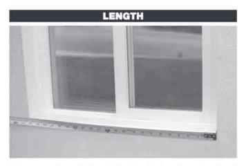
Measure the width of the inside jamb to jamb of the window opening.
